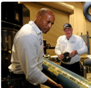
out of the aquifer, a layer of rock and sediment deep under the ground, and treated at the Arlington Desalter through a process called reverse osmosis, which forces water across a membrane at high pressure. The membrane traps salt and other impurities and allows only clean water to come through, allowing us to drink the water.
